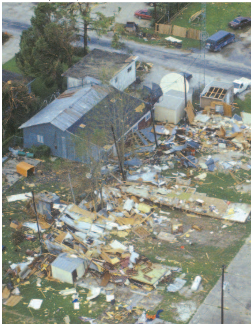
Aerial view of damage caused by Hurricane Andrew.
